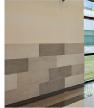
TILE - WAINSCOT INSTALLATION IN CORRIDORS
